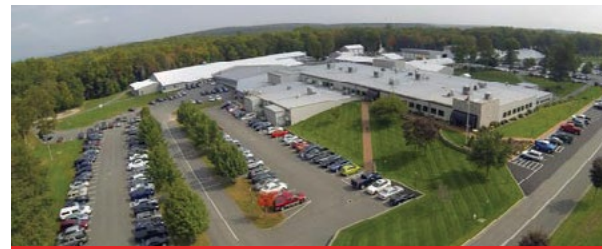
Chester, Connecticut facility
